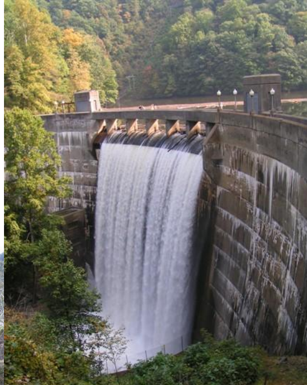
Pinnacles Hydro, Virginia, USA
